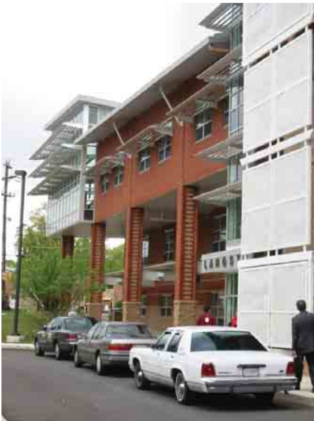
Simple additions to the building envelope, including louvers for windows, will help reduce energy consumption for building heating and cooling.
