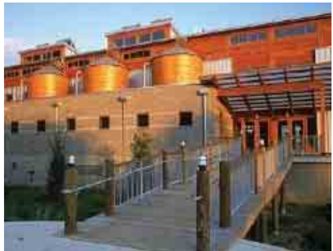
Rain cisterns on this LEED Certified Platinum building in Maryland are used to store stormwater on site for re-use.
