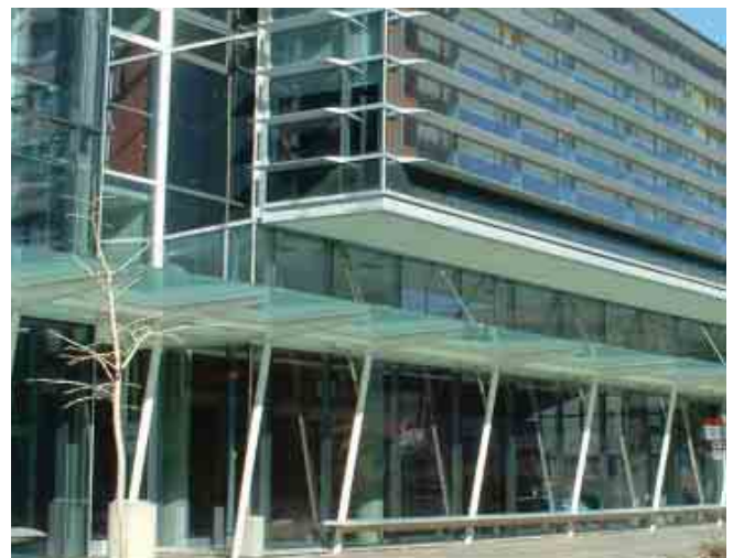
Transparent covered walkway integrating pedestrian seating.
