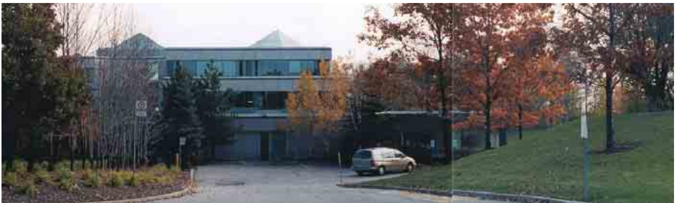
Examples of building typologies appropriate for the Business Park - Natural Heritage Oriented Areas.
