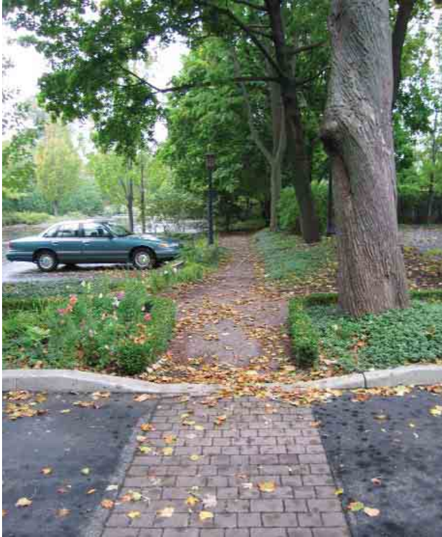
Pedestrian walkway paving should differ in material and appearance from vehicular routes.
