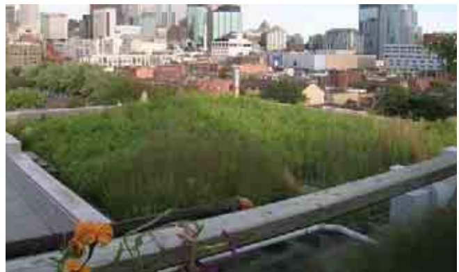
Wherever possible, bioswales and green roofs should be incorporated in addition to end-of-pipe stormwater management facilities.
