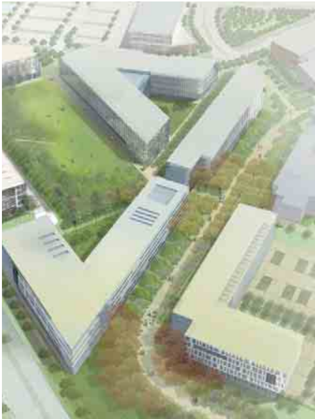
The Derry Green Corporate Business Park will feature both street oriented and campus-style layouts. The above example illustrates a campus type development.
